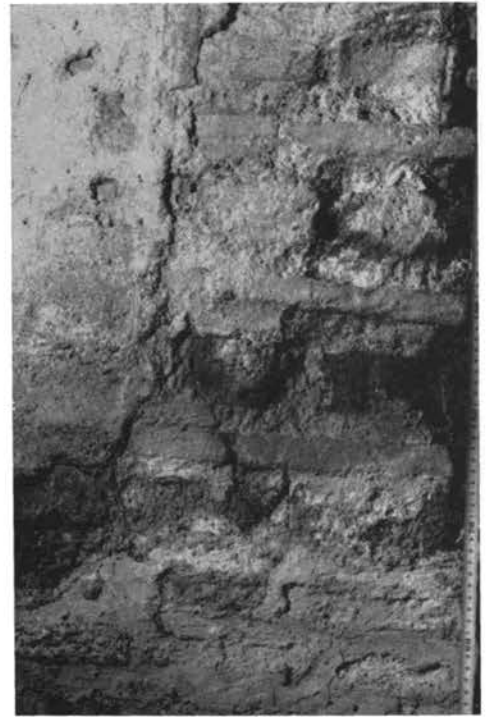
Fig. 89b. S. Martino ai Monti, Roman Hall, opus listatum blocking doorway to building P
